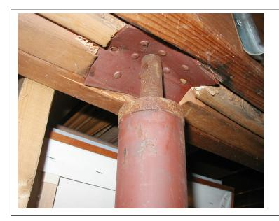
Inadequate spreader plate on top of a screw column, the plate is crushing into the main beam, a Failure.
