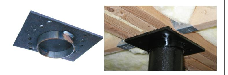
Referred by some as a Springfield spreader plate, it is thick and as wide as the beam, twice as long as wide. it will not bend, it spreads the load well. Holes are to secure the plate to the beam which is required. An installed Springfield plate, note spans entire width of main beam.
