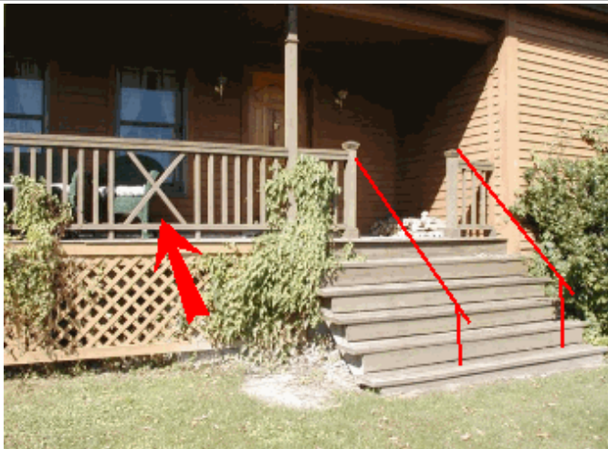
Add handrails along steps and openings below handrail too large in areas
