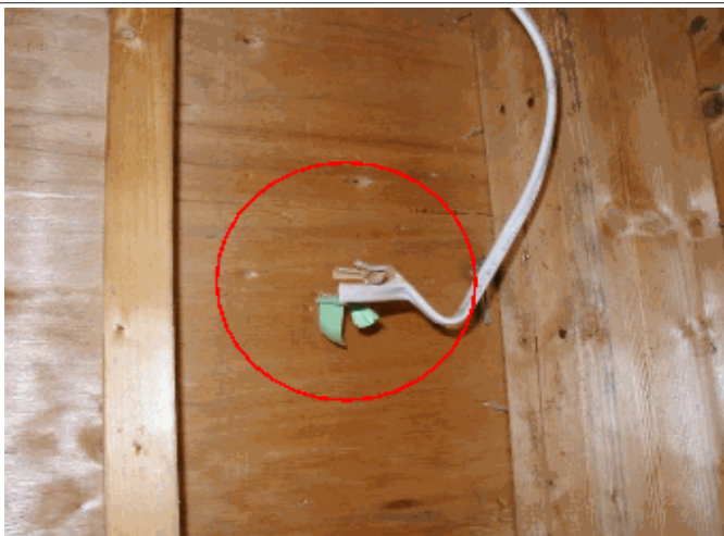
Elect.: Terminate free end wires in boxes, this one in garage & one in master bedroom
