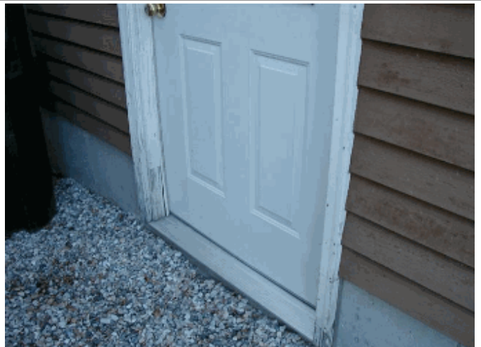
Exterior: Paint trim on garage door to avoid wood rot
