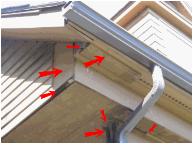
Exterior: Missing molding outside
