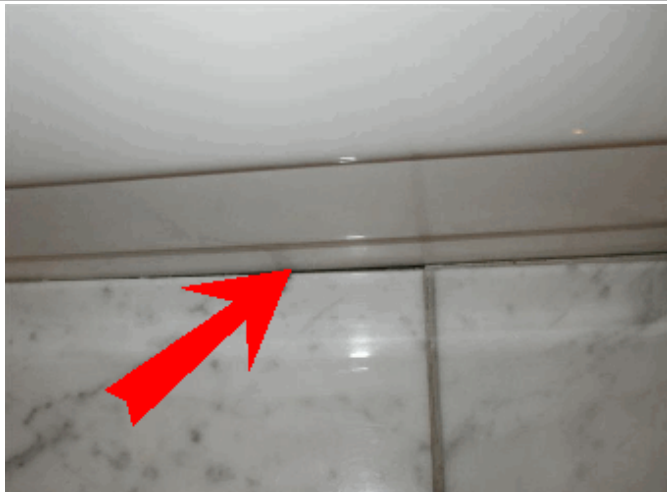
Seal between tiles and tub/showers
