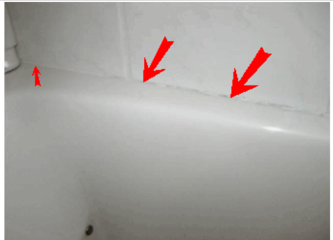
Seal between jet tub and walls
