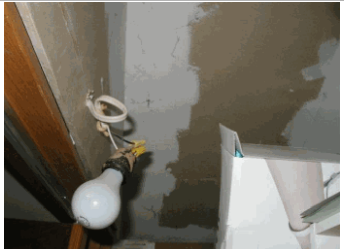
Bedroom closet has unsafe light, is a fire hazard, install pertinent fluorescent light
