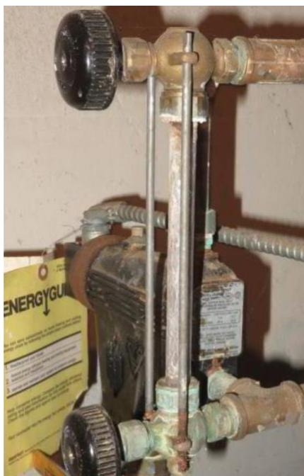
This is a very dirty sight glass that needs to be replaced. Note the white color around the nut at the top of the sight glass and the white color on the outside, water has been leaking out the seal at the top of the glass and possibly out the bottom.
