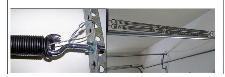
The left photo shows a steel cable secured at one end and entering the tension spring. The other end of the steel cable needs to be secured as well, to properly retain the spring when it breaks.
