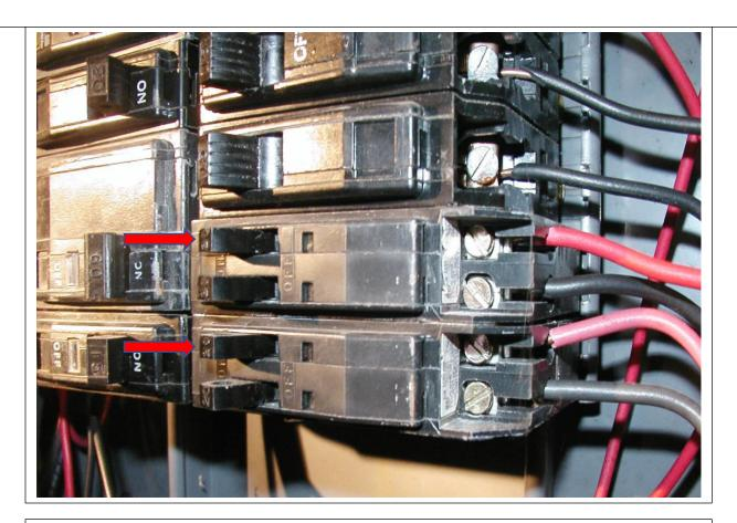
Above are two tandem breakers, they are double breakers that fit where usually only one breaker does. They are actually two separate breakers, but they are on the same leg of power. So, in this case the tandem breakers that feed a multi wire branch circuit can overload the neutral.
